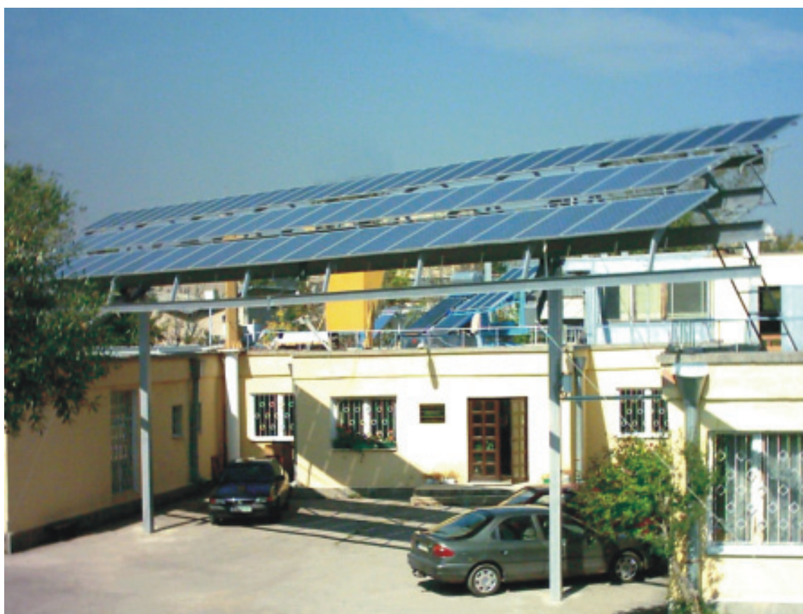
Fig.1. A view of the PV module supporting and tracking system
