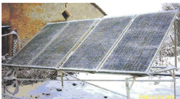
Denima 2001 create a Photovoltaic station supplying the street lighting in Gorno Osenovo village on 1000 m height in Pirin mountain.
