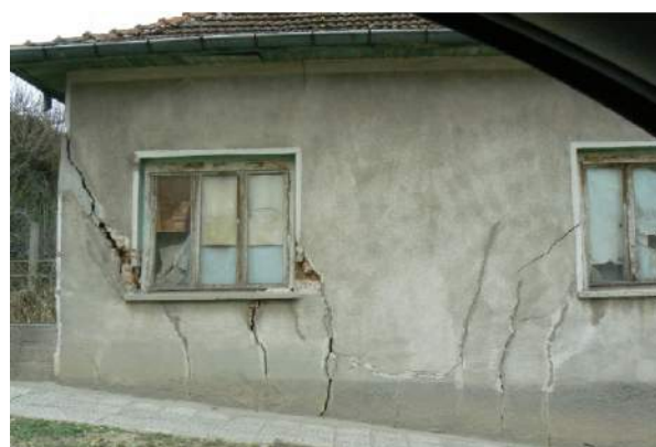
Figure 5. Damaged house by landslide Gorni Vadin Village, March 2013
