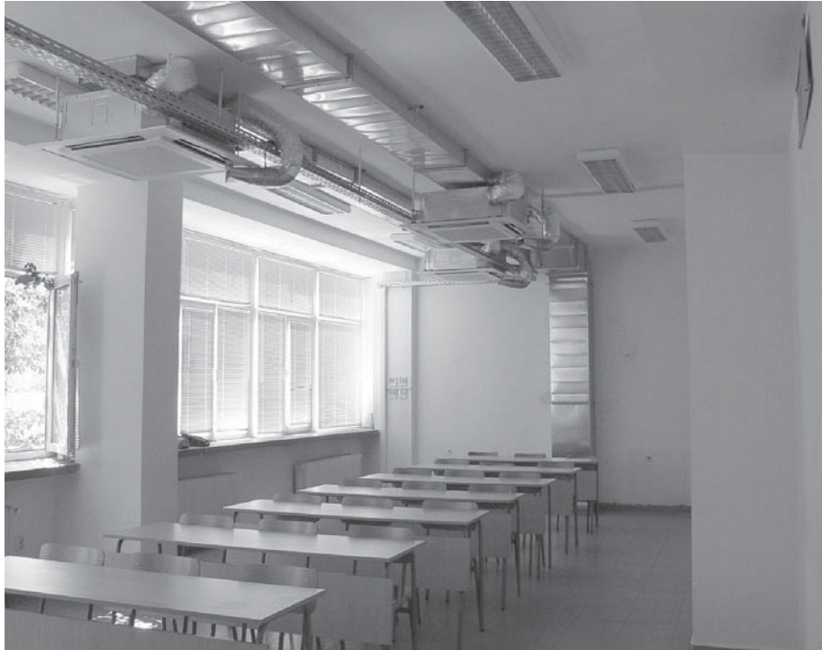
Fig. 8. Left side view of the established laboratory with the installed equipment
