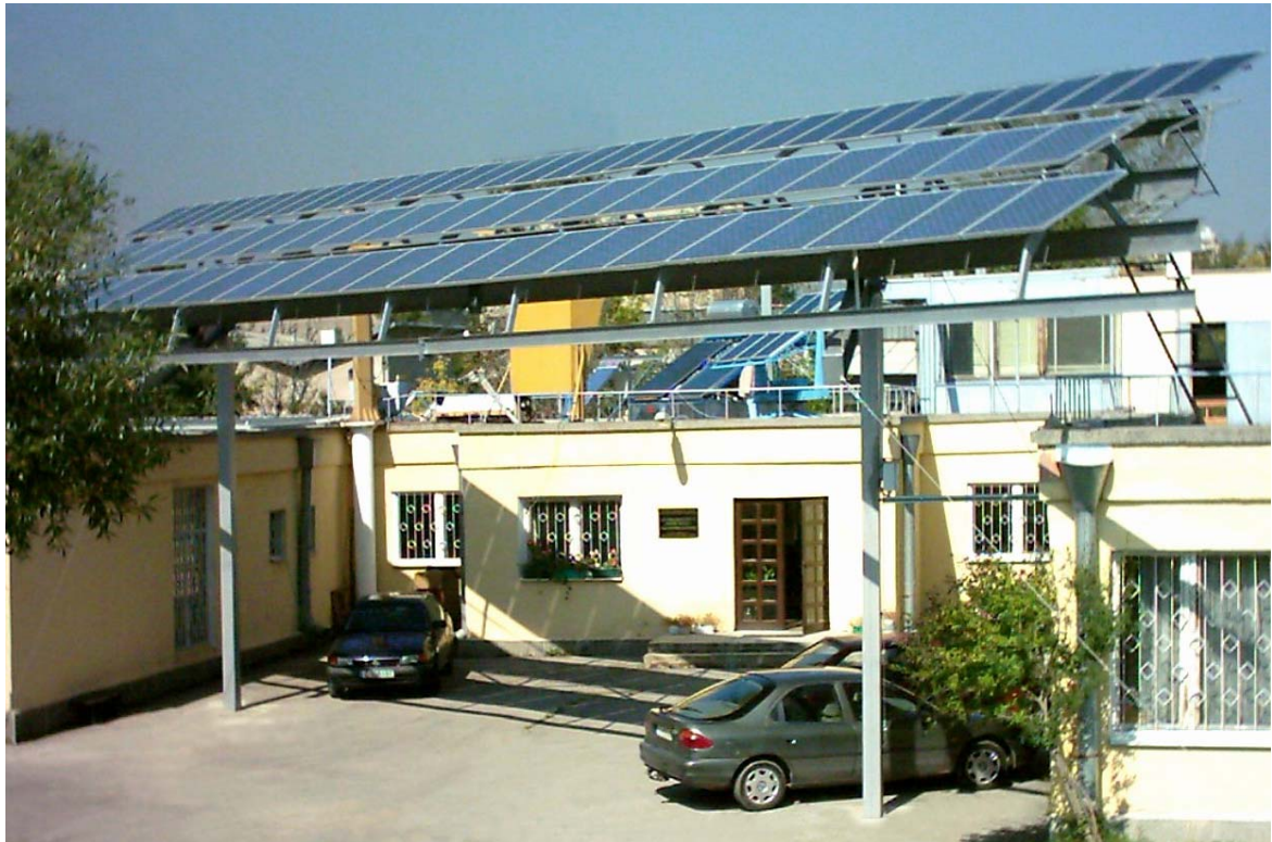
Fig. 1. A view of the PV module supporting and tracking system
