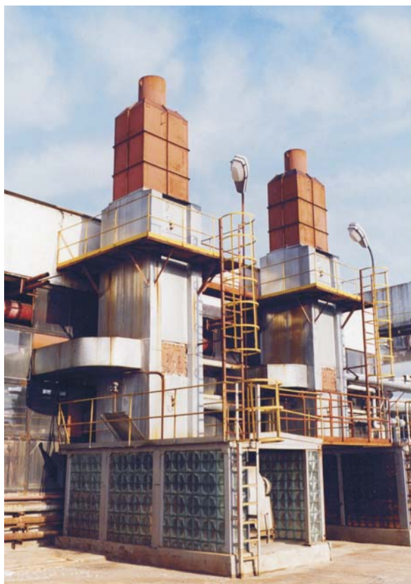
Fig. 2. Second generation contact economizers in the district heating station Plovdiv South.
